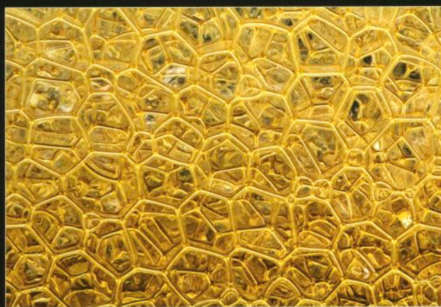
The exterior of the Beijing National Aquatics Center (top) is based on the Weaire-Phelan structure, formed by repeatedly joining two different shapes of equal volume to minimize their shared surface area. The interior of the building (middle) shows the polyhedral structure more clearly. A very coarse foam (bottom) looks strikingly similar.
